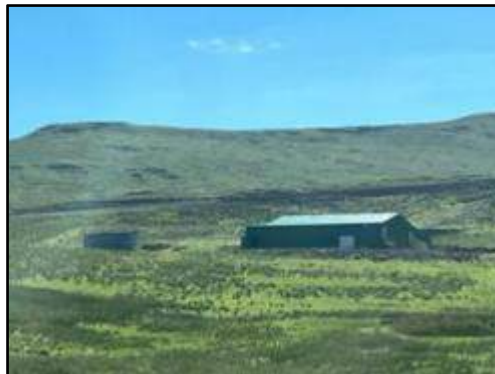
Figure 3- 5 Shearing shed at Semenanyane Iketleng
