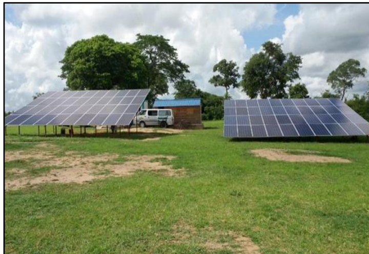
Figure 1- 3: Solar PV array 3
