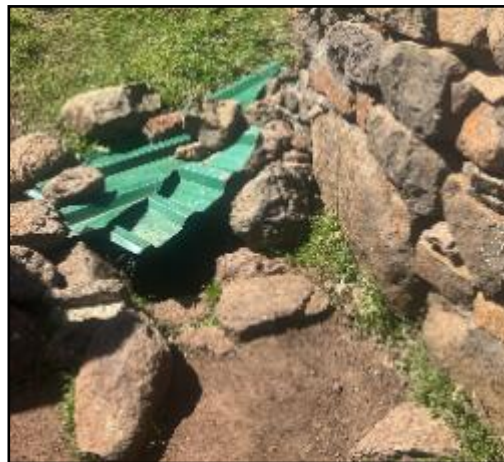
Figure 3- 3: Unprotected well at Masaleng
