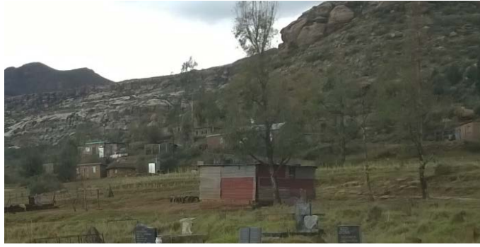
Figure 19: Temporary Structure (photo: David Fernandez)
